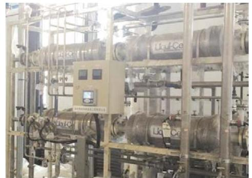
3M™ Liqui-Cel™ EXF-10x28 Series Membrane Contactor
